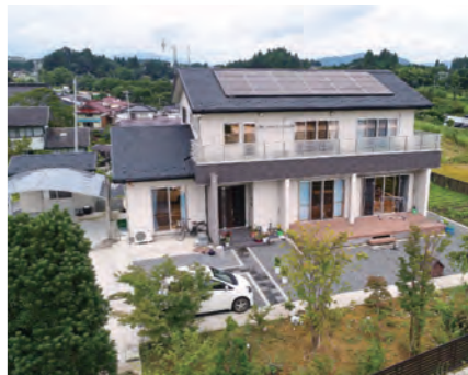
●K様邸新築工事
